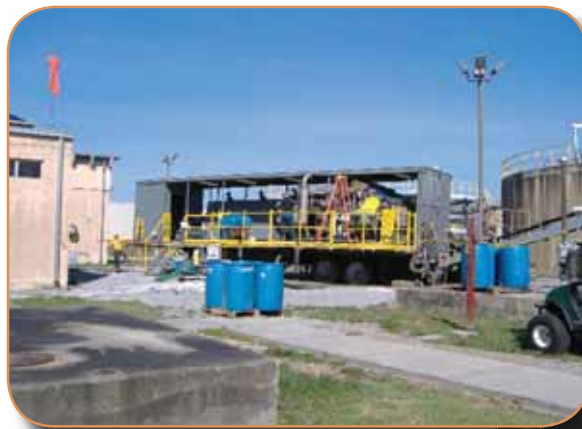
South Wastewater Treatment Plant
