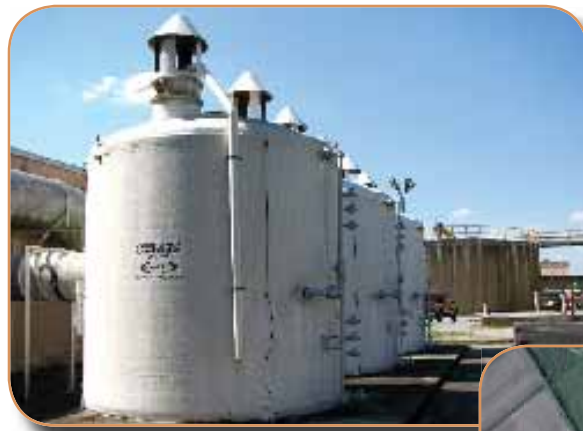
South Wastewater Treatment Plant
