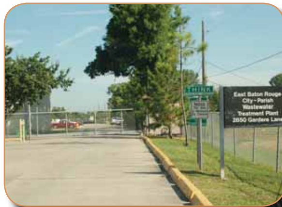
South Wastewater Treatment Plant
