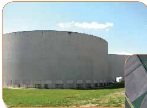
South Wastewater Treatment Plant
