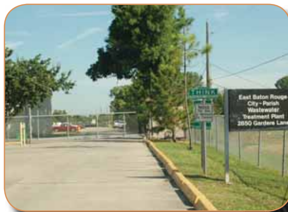
South Wastewater Treatment Plant
