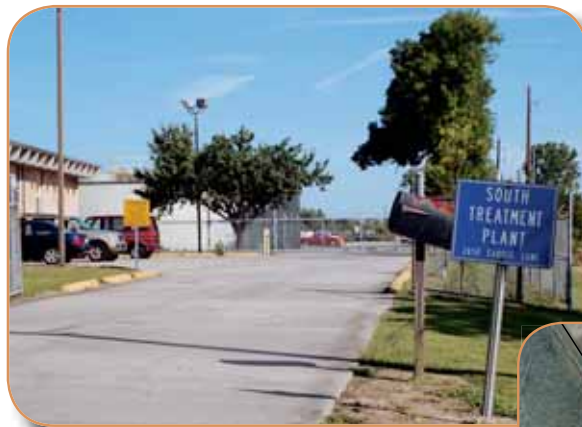
South Wastewater Treatment Plant
