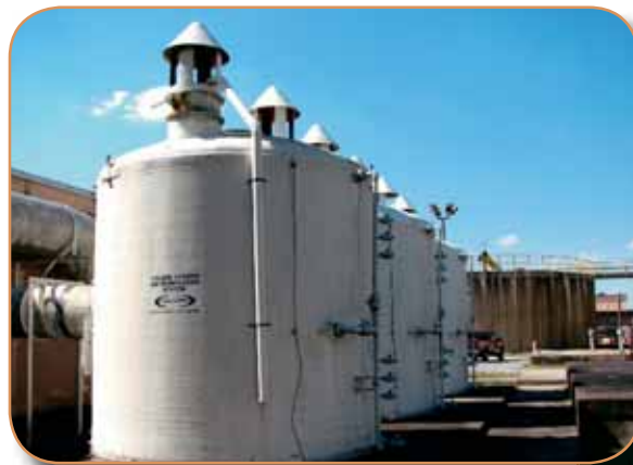
South Wastewater Treatment Plant
