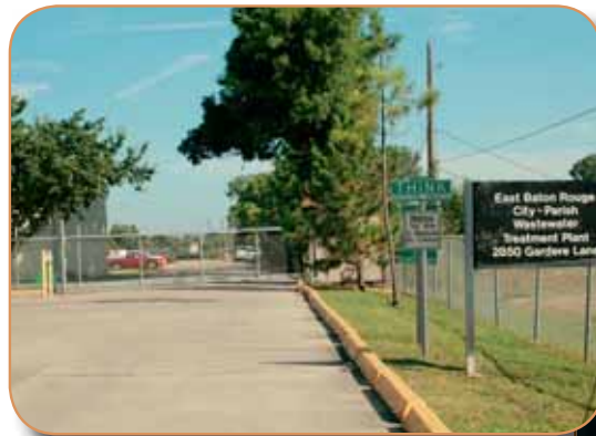
South Wastewater Treatment Plant
