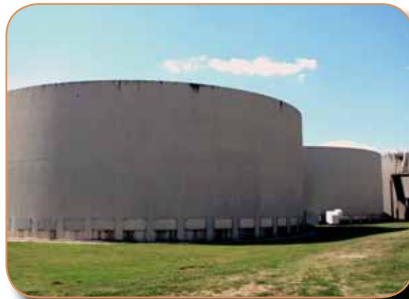
South Wastewater Treatment Plant
