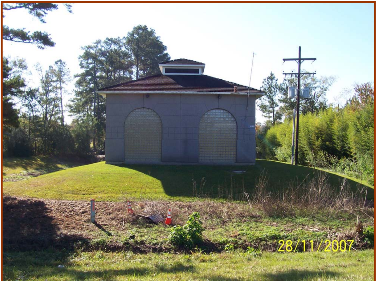
Booster Pump Station 511 is on Hooper Road approximately 1.1 mile east of Foster Road
