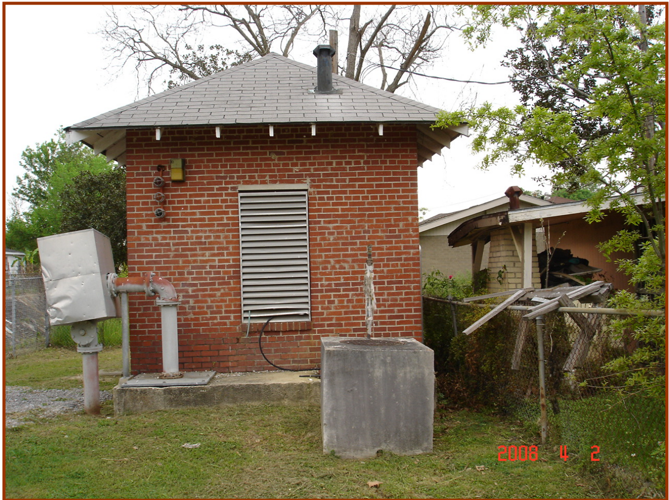
This project involves upgrading PS15, which is located along Washington Street, south of the intersection of Washington Street and West Belfair Drive
