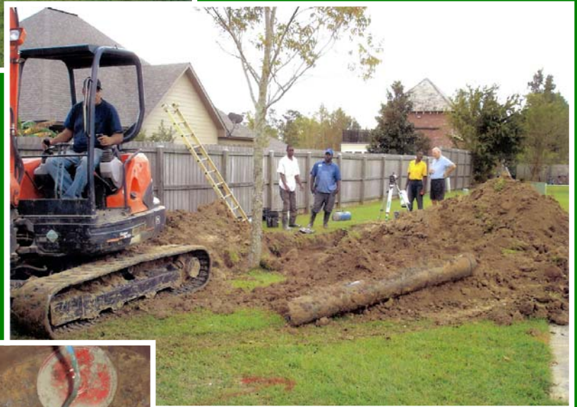
One of the first steps in rehabilitation includes a manhole inspection.
