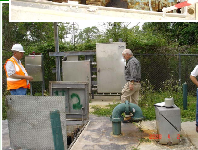
The PS136 Area Upgrade project is located in the Lake Sherwood Acres area and consists of the demolition of nine existing pump stations, including PS136, which will be upgraded including approximately 2,000 feet of forcemain.
