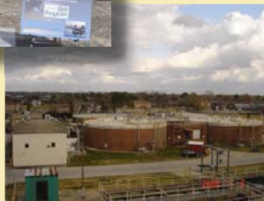
Several improvements will be made to the SWWTP
