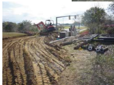
Looking North of the Santa Maria Golf Club, the existing pump station 382 is being readied for the replacement of its pumps with two new 150hp pumps.
