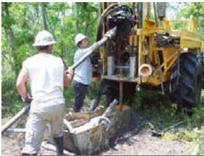
Geotechnical Engineers are drilling soil samples in the Northwest Area of the SWWTP. Results of the soil samples will be used to help assess the site characteristics where the proposed Equalization Tanks will be constructed.
