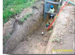
Trench boxes are used for the gravity line installation in the Comite – Foster Area.
