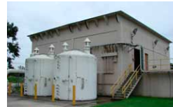
Odor problems will be reduced in the North WWTP.
