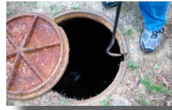
657 manholes will be inspected in the Staring Lane area.
