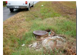
775 manholes will be inspected in the Scotland Avenue – Progress Road Area
