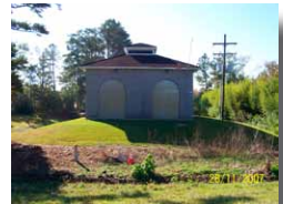
The forcemain near Booster Pump Station 511 goes down Hooper Road approximately 5,700 linear feet.
