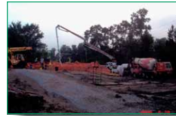
Construction at PS136, a 4.5M gallon per day pump station, continues.
