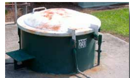
Pump Station 230 will be replaced in the Sullivan Road area.
