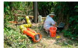
200,500 linear feet of pipe is inspected in the Gardere – Burbank area.
