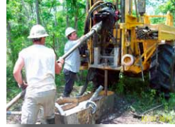
Geotechnical investigations begin conducted at the SWWTP.
