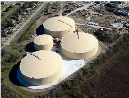
Aerial of Storage Tanks
