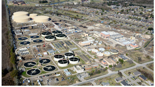
South Wastewater Treatment Plant
