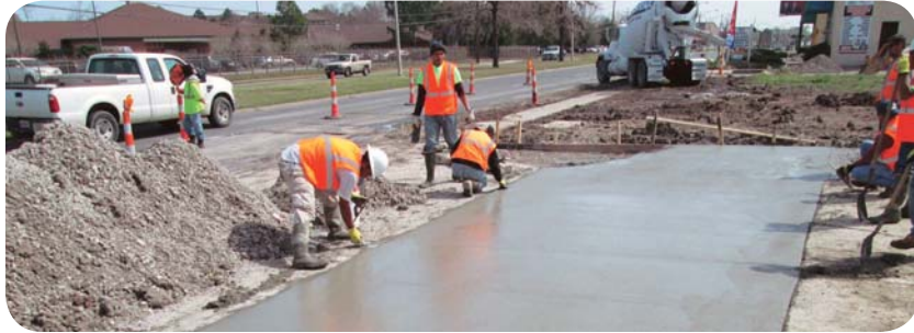
Road restoration includes laying concrete, as exemplified in the picture above.
