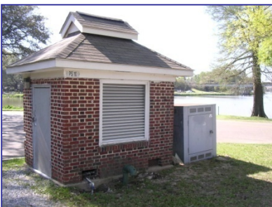
Pump Station #10, East Lakeshore Drive, near southeastern corner of City Park, will be upgraded.
