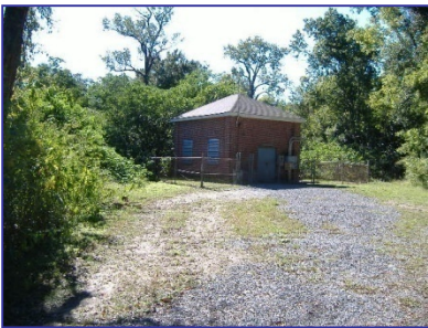
Pump Station #3, located at Acadian Thruway, near Bawell Street, will be upgraded.
