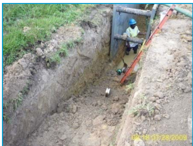
Trench boxes are used for pipeline installation.
