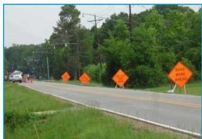
Signage notifies residents of underground construction activities.
