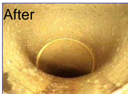
Simply cleaning the pipes and manholes in preparation for the physical inspection removes blockages, debris and roots.
