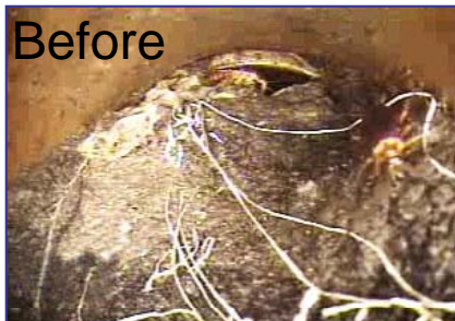
Simply cleaning the pipes and manholes in preparation for the physical inspection removes blockages, debris and roots.
