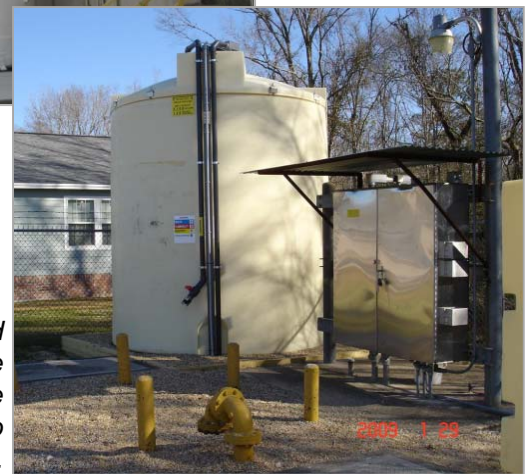
Chemical feed systems were installed at five pump stations to reduce odor.
