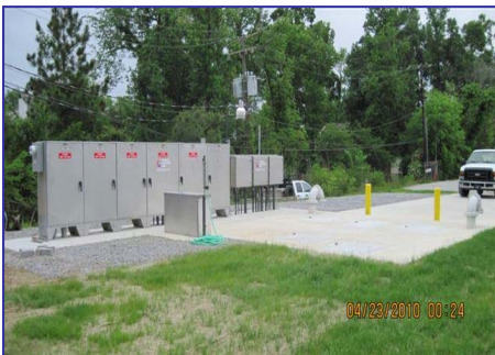
Pump Station 136 finished.
