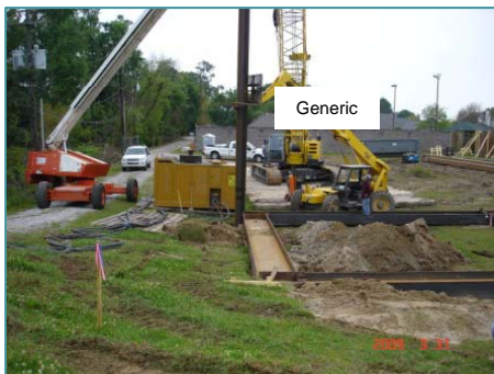
Installing the new wet well for Pump Station 136
