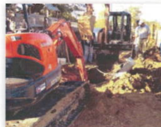
Rehabilitation construction continues in the Round Oaks Subdivision.
