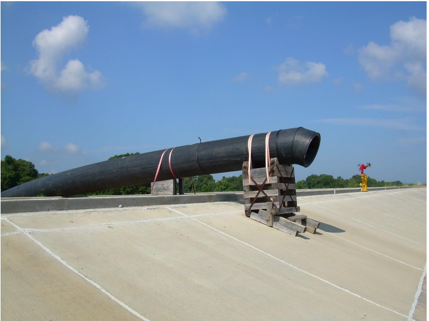
Figure 5. Temporary recirculation above-ground HDPE piping installed to facilitate pump station testing
