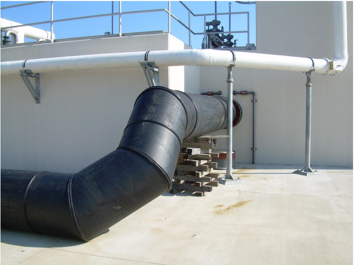
Figure 3. Temporary recirculation above-ground HDPE piping installed to facilitate pump station testing
