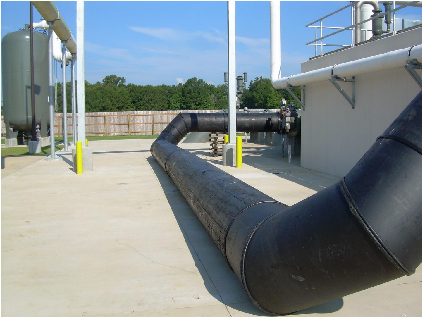
Figure 4. Temporary recirculation above-ground HDPE piping installed to facilitate pump station testing
