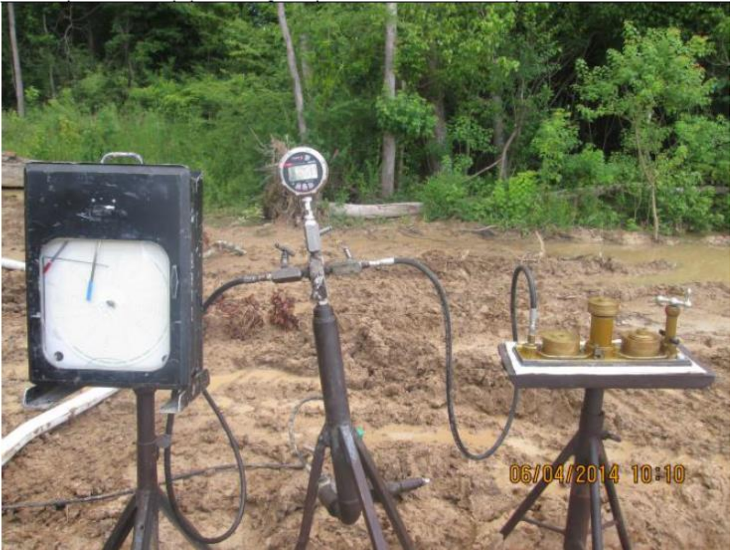
Figure 6. Pressure testing of sanitary sewer forcemain
