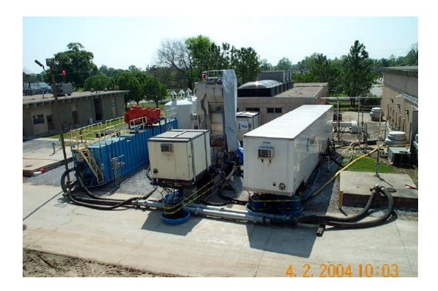
The above photo shows the ballasted flocculation pilot testing equipment located at the SWWTP. Starting from the left, the first unit is a storage/mixing tank utilized by both sets of equipment, the middle unit is the DensaDeg equipment and the unit to the right is the Actiflo equipment. Behind the equipment is bar screen building, to the left is the administration building, and to the right is the influent pump station building.
